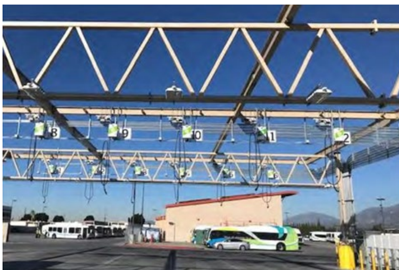
Figure 4. Overhead Plug-in Charging Example (Source: Burns McDonnell Foothill Transit In-Depot Charging and Planning Study)
