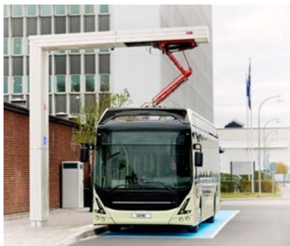
Figure 7. On-route Overhead Charging (Source: ABB)
