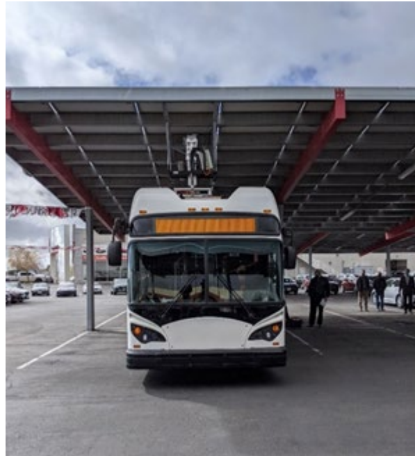
Figure 5. In-Depot Overhead Charging Example (Source: CALSTART)
