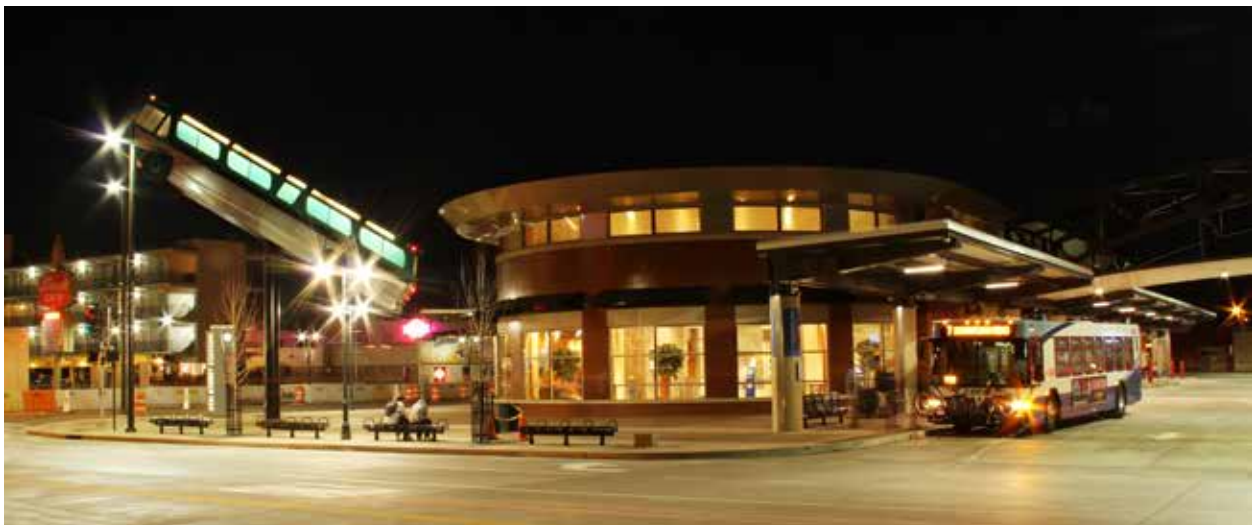
Regional Transportation Commission - 4th Street Transit Center
