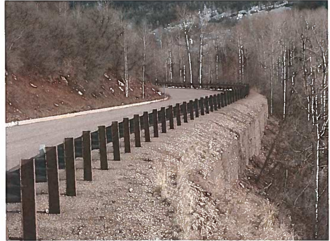
Photograph 2. Cast in Place Concrete Wall
