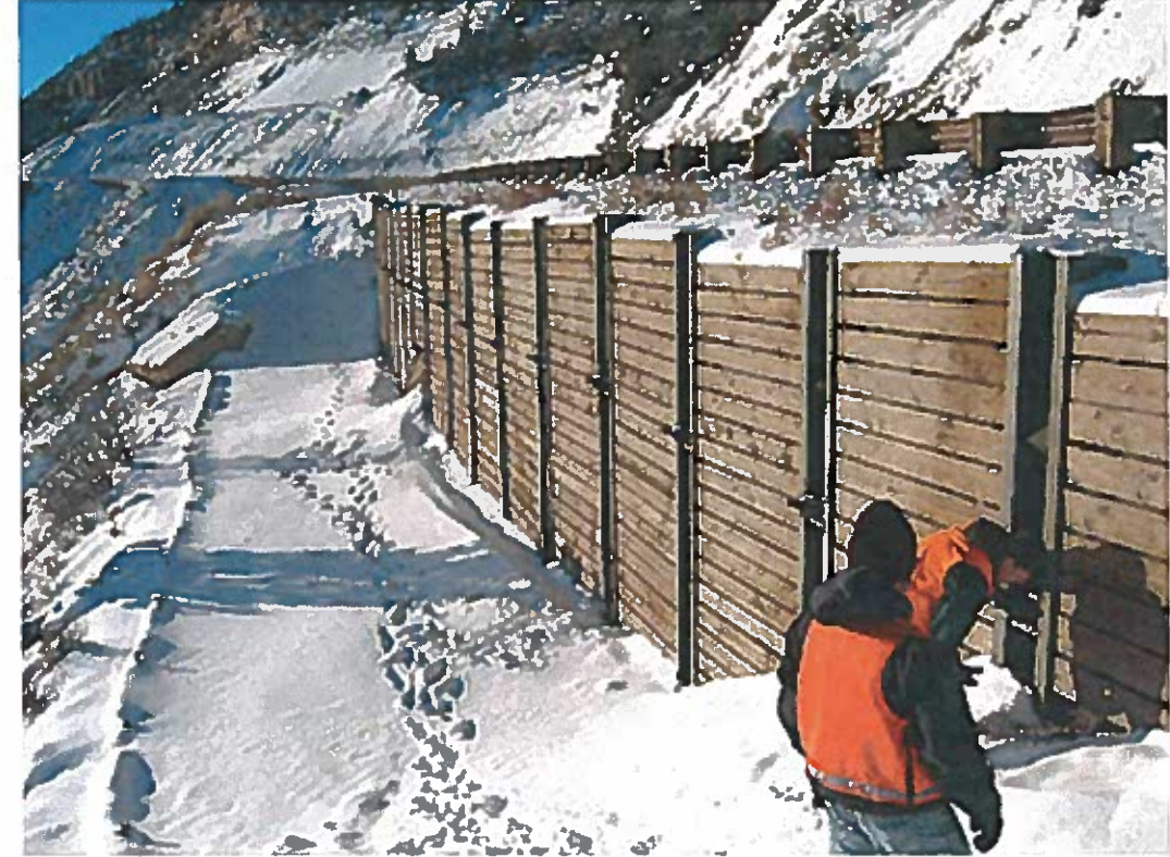
Photograph 6. Soldier Pile Wall with Timber Lagging
